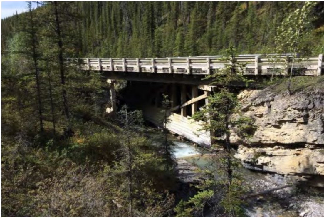
Peterson Creek Bridge No.2
